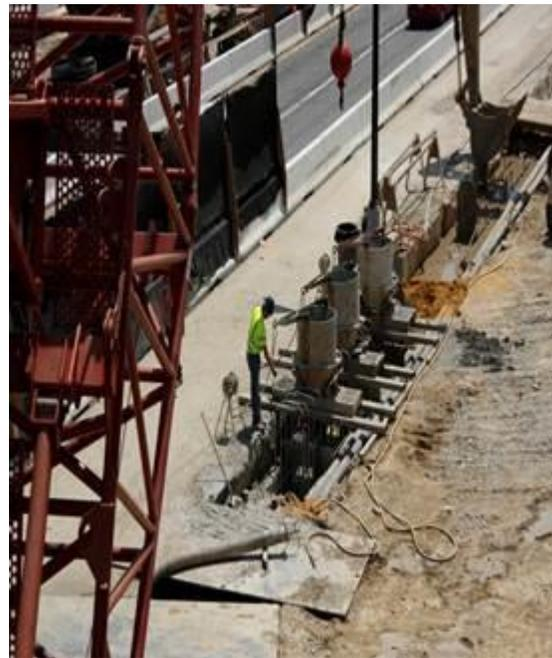
Concrete being pumped into the slurry wall
