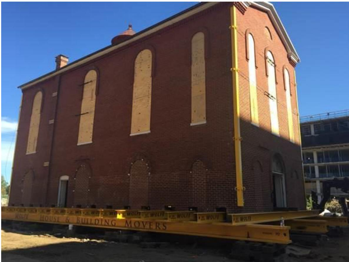
the three main beams and all of the crossbeams have been set. Yellow metal supports have been placed at the four corners of the building and cables that surround the building will soon be tightened to compress the walls so that the bricks don't shift as the building is lifted from its foundation. The building will be lifted off its foundation on October 31. The move will take place around 10:00 a.m. on November 3.
