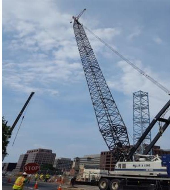
The 200-Ton Mobile Crane That Built the Tower Crane
