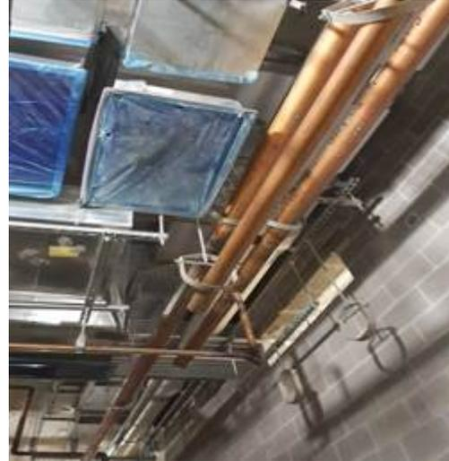
variable air volume (VAV) boxes that control the flow of air for heating and ventilating are being connected by ductwork that lines the ceilings on each floor. And in the construction trailers, the architects, engineers, construction managers, and subcontractors continue to review drawings, make field adjustments, rethink design to meet constructability contingencies, and coordinate the various internal and external systems so that the building comes together as originally conceived.
