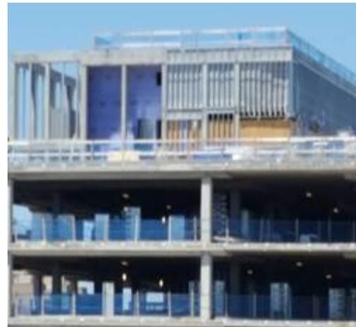
in. Anchors for the windowed curtainwall have been installed on the slab edges; when you return in the Fall, you will see the building substantially enclosed.
