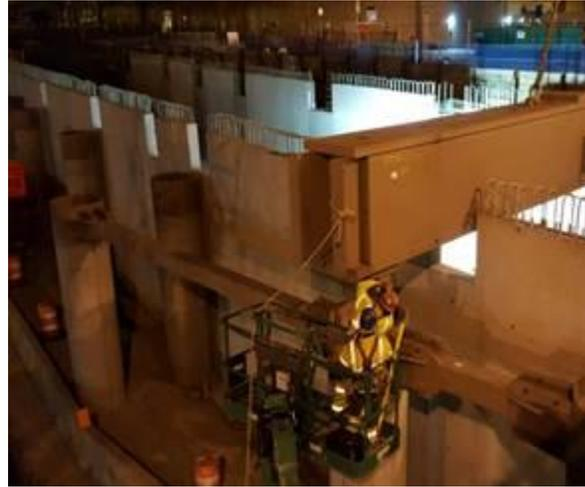
onto narrow pins that rise from the columns to hold the beams in place. Once the beams settle in, workers mount the girders and fasten the bolts that hold the girder to the column, thus ending an industrial ballet, choreographed to create the structural support for the platform.
